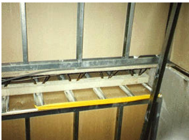
Electrical cables for stair lighting. (A steel stud stands leaning against the corner)
